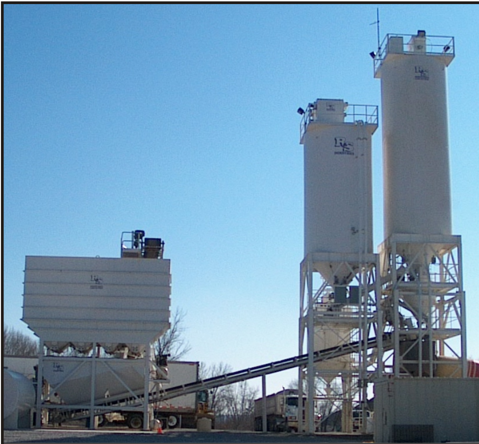
Apache Batch Plant 943 Arrowhead Silo & 720 Auxiliary Silo
