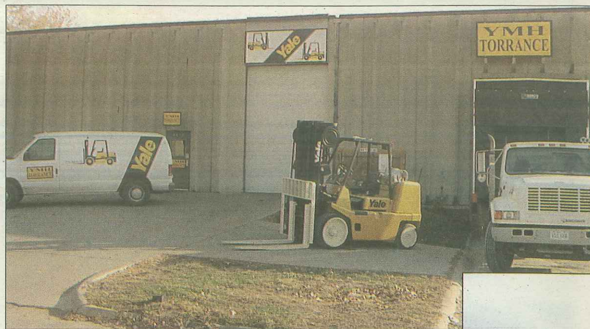
LEFT: The YM-H Torrance office in Des Moines was added to the company in August of 1998. With this addition the company can better serve its clients because of its increased rental ability, well stocked parts inventory at each location and a larger service department to keep fleets running.
